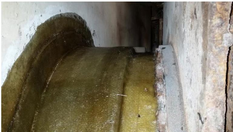
First stage has been applied. When cured, this stage provided a sound surface over pipe and concrete to support lamination.
