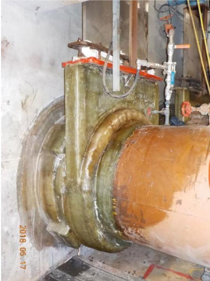
Installation of laminate on the force main pipe and valve
