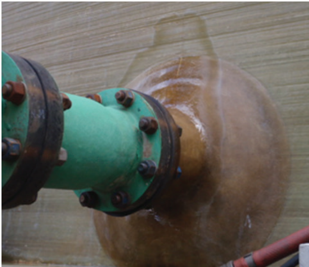
Figure 8. Cracks and leaks in the outer surface that require corrective action.
