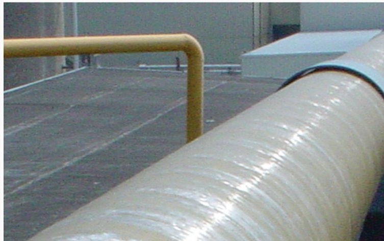
Figure 11. Exposed reinforcement where corrective action is required.
