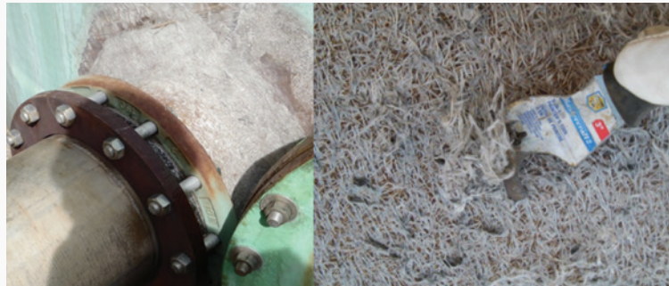
Figure 10. Reinforcement where no corrective action is required.
