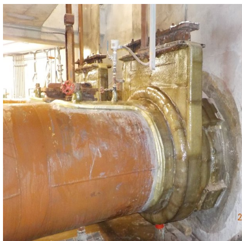
Figure 4 Installation of laminate on the North and South force main pipes and gate valves
