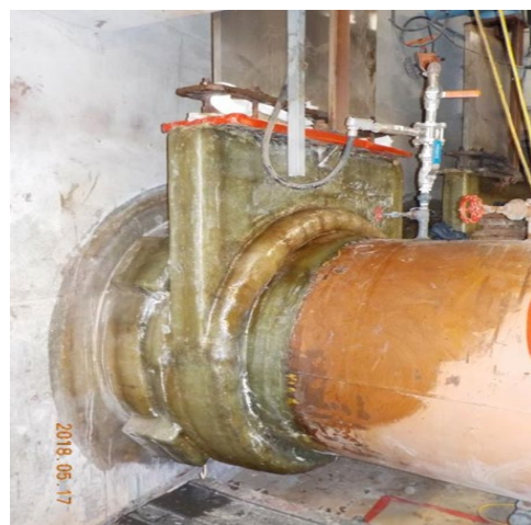
Figure 4 Installation of laminate on the North and South force main pipes and gate valves
