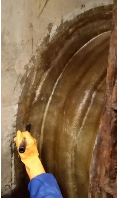
Figure 2 Applying FRP stages
