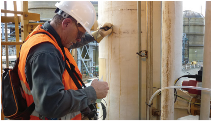
Figure 5. Non-Intrusive FRP Inspection
