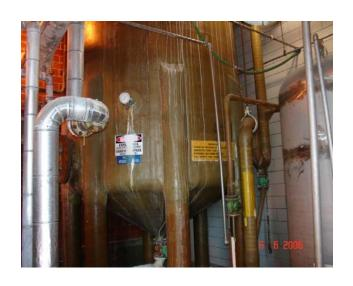
Service: Chlorine dioxide, bleaching stock, sodium hypochlorite, chlorate, bleach filtrates, wastewater, etc
